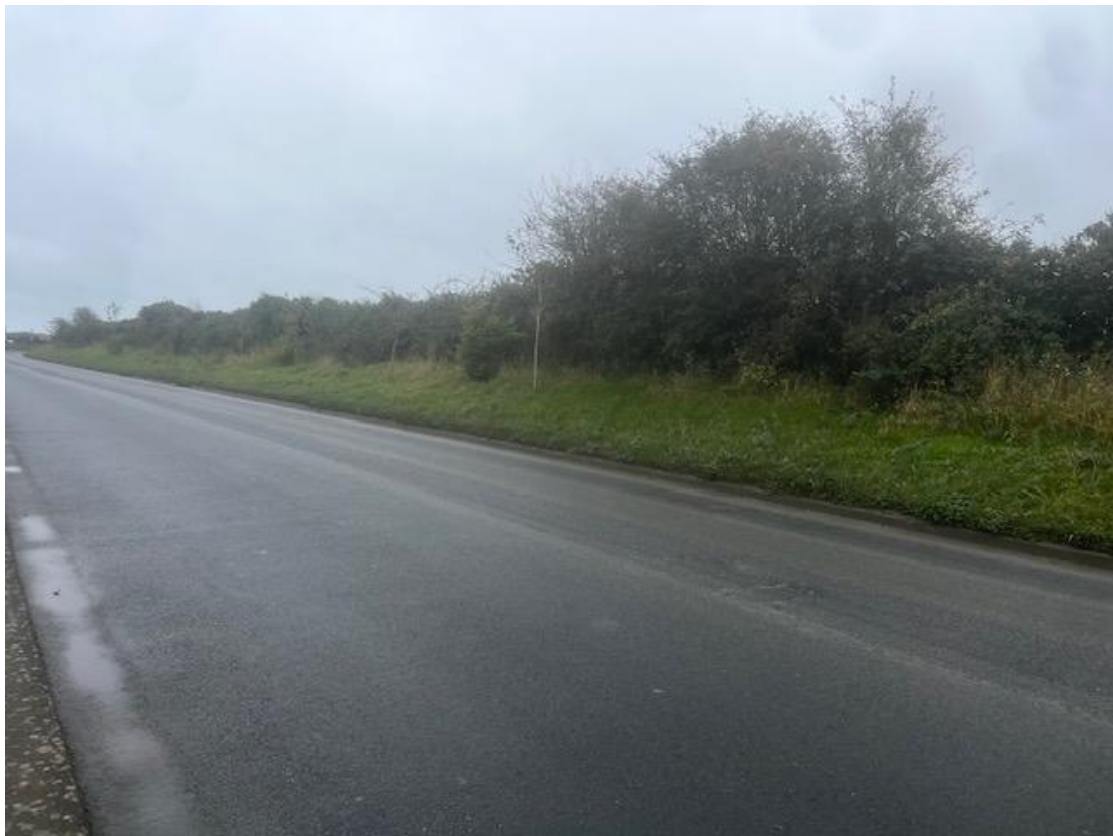
Plate 7-1 Conduct regular maintenance to prevent overgrowth
